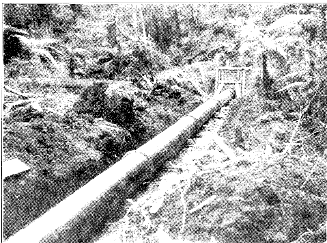
Round Hill Mining Company. Penstock at head of Pipes.
