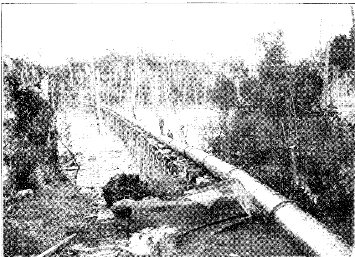
Round Hill Mining Company. Continuation of Pipes to supply Elevators.
