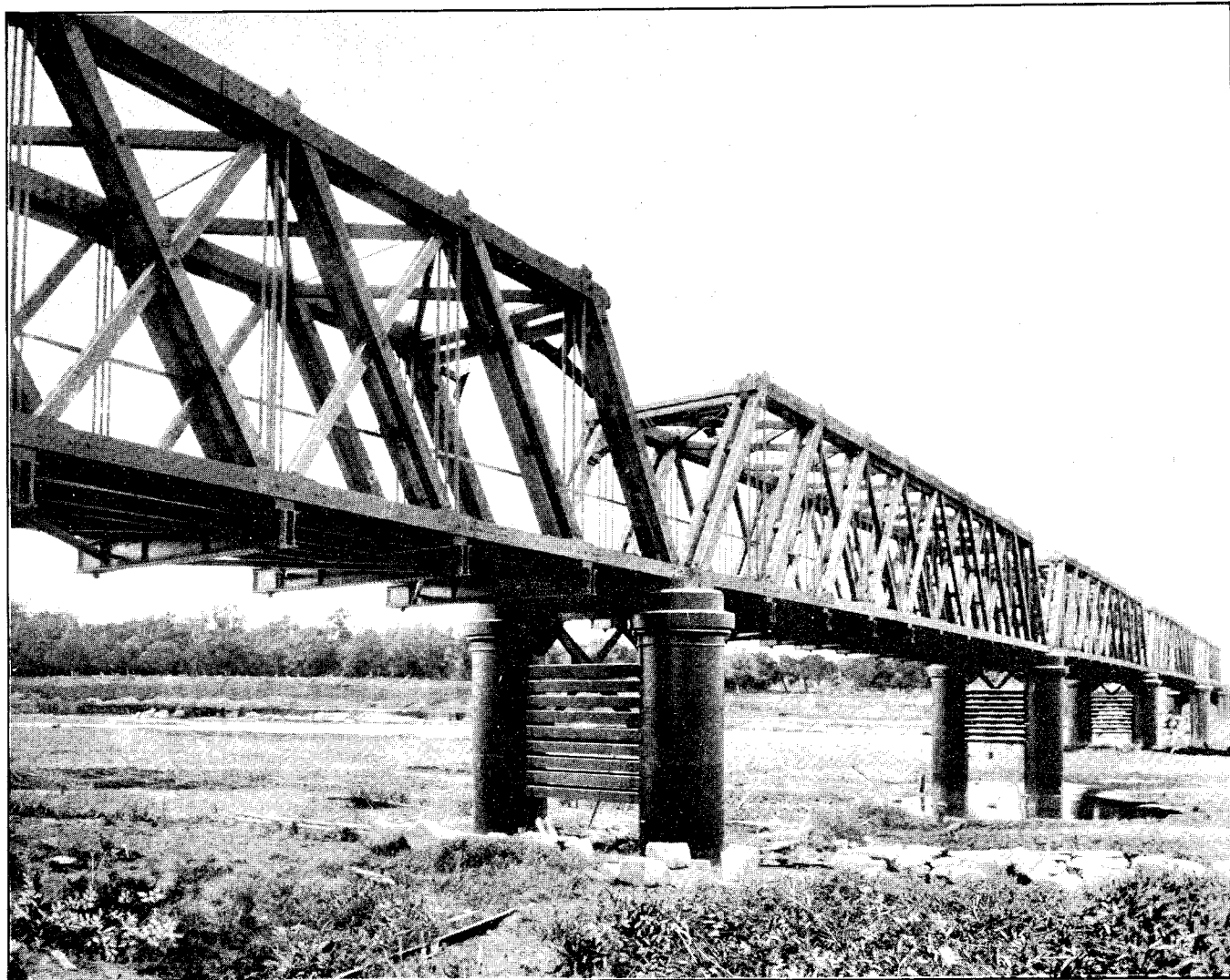
Rangitikei Road and Railway Bridge, 5 spans, each 120 ft.
