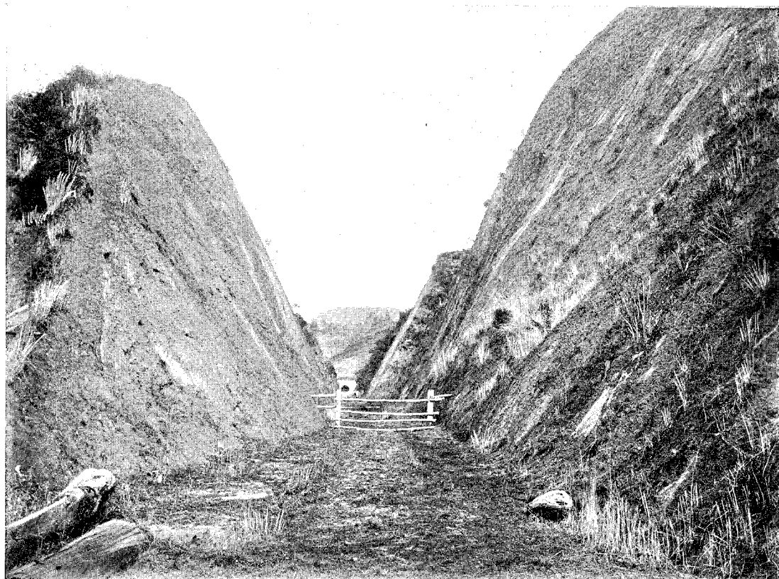
North Island Main Trunk Railway, Mangaweka Section—A Papa Cutting.
