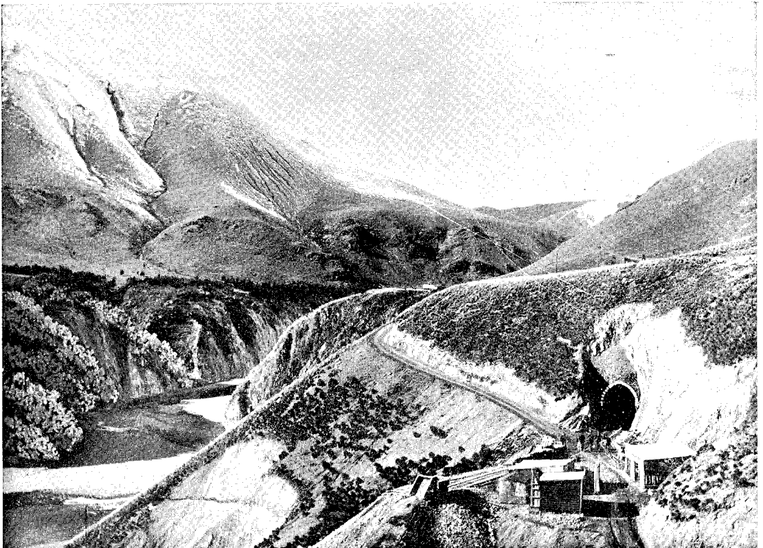
Midland Railway, Springfield End—Tunnel Front at 8 m. 75 ch., and Service Road giving access to Works.
