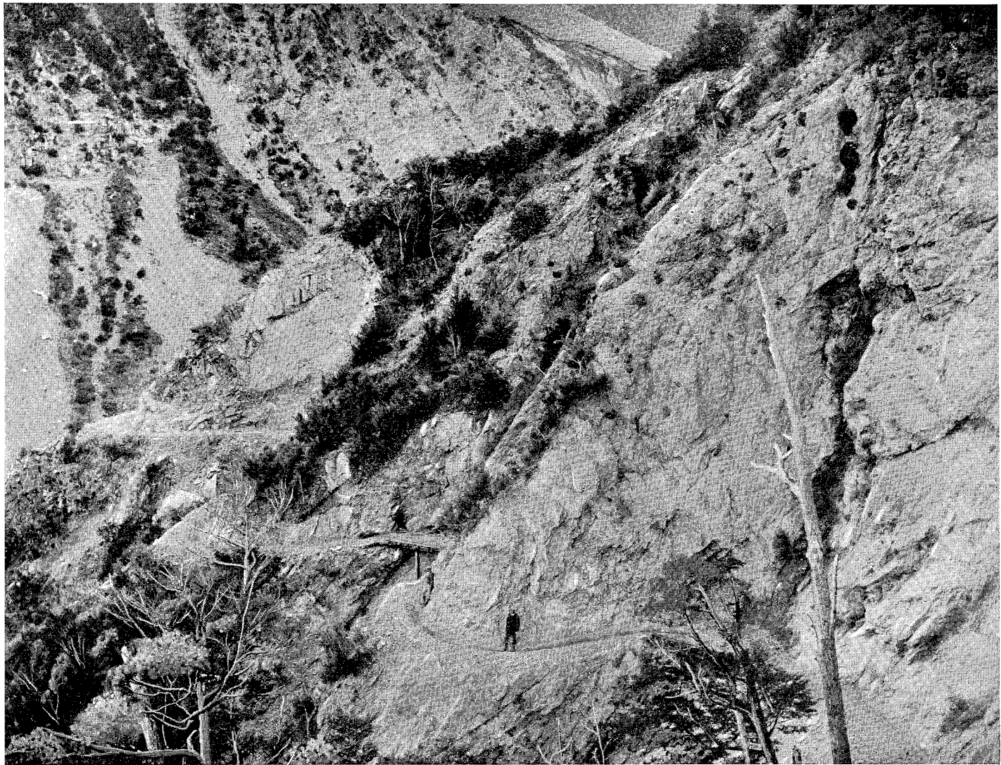
Midland Railway—Service Horse-track over Staircase Gully.
