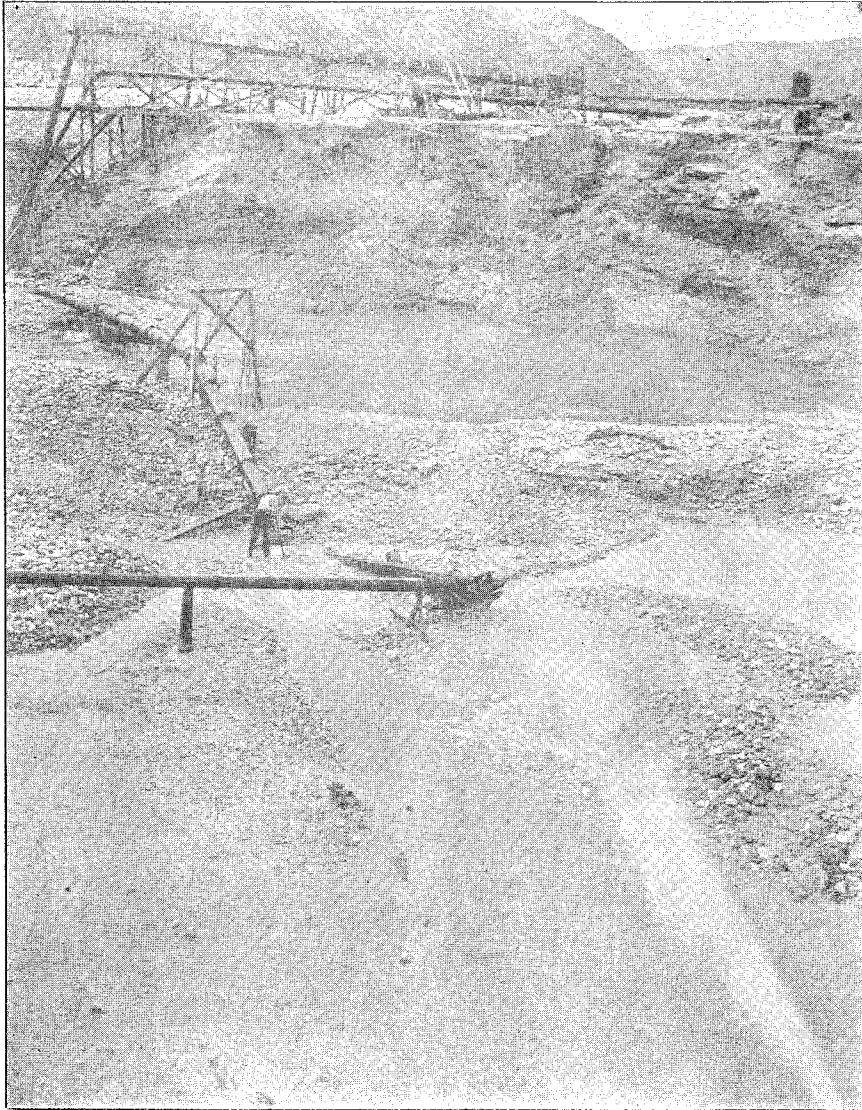
Champion Hydraulic Company's Claim, Beaumont, Otago, showing means adopted to convey alluvial wash from low dip to Main Elevator. C. 3.
