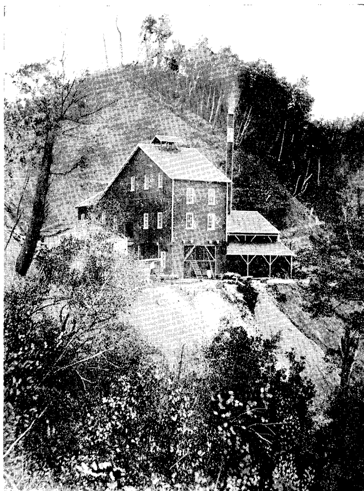
Progress Mines of New Zealand: "B" Shaft house.
