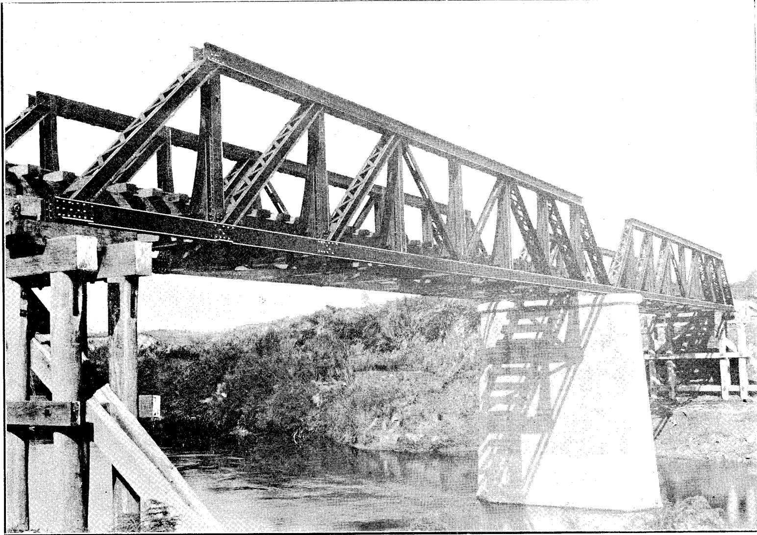
North Island Main Trunk Railway.—Ongarue River Bridge (No. 2 Crossing). Three 30 ft. and two 80 ft. spans. Height from river-bed to rail-level, 37 ft.
