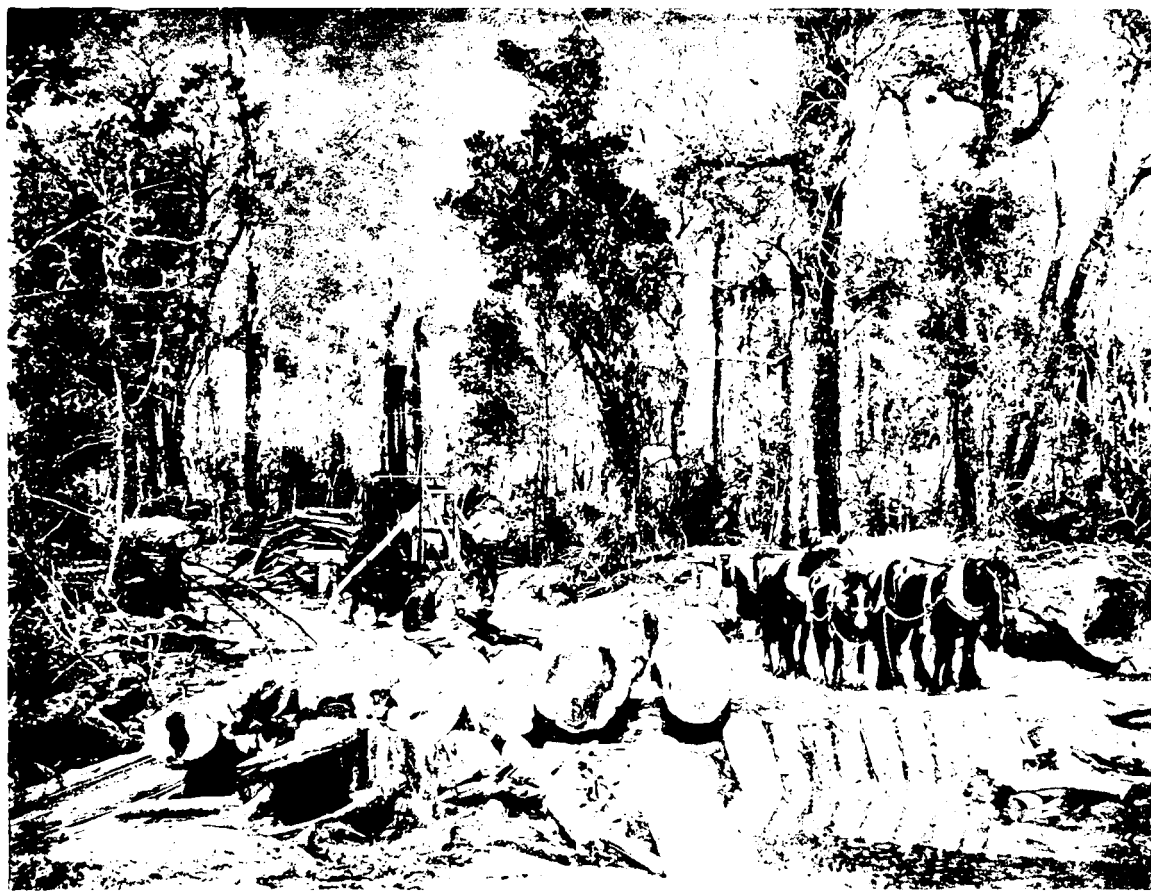
3. LOG-HAULING, RONGA VALLEY, MARLBOROUGH.
