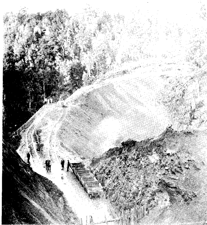
NORTH ISLAND MAIN TRUNK RAILWAY. 110 FT. BANK ON SPIRAL.
