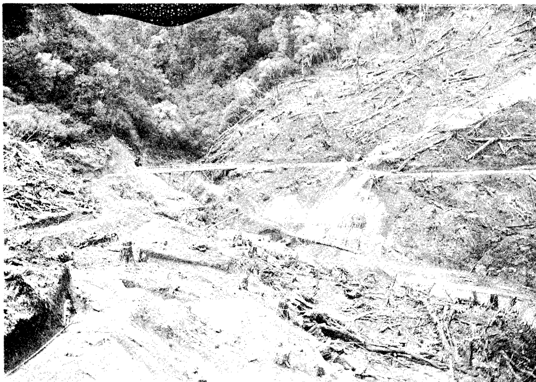
NORTH ISLAND MAIN TRUNK RAILWAY. HAPAAWHENUA VIADUCT (1ST OCTOBER, 1907).
