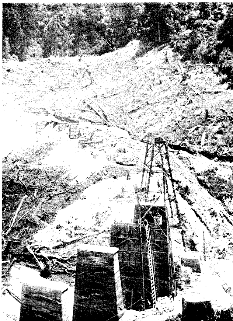
NORTH ISLAND MAIN TRUNK RAILWAY. HAPAAWHENUA VIADUCT (ABOUT CHRISTMAS, 1907).
