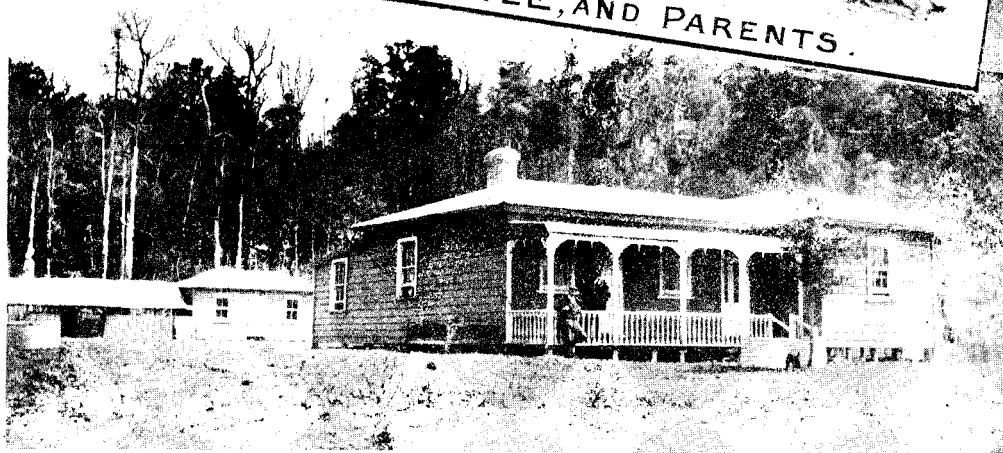
HOUSE BUILT AFTER PLAN OF N.S. RESIDENCE.
