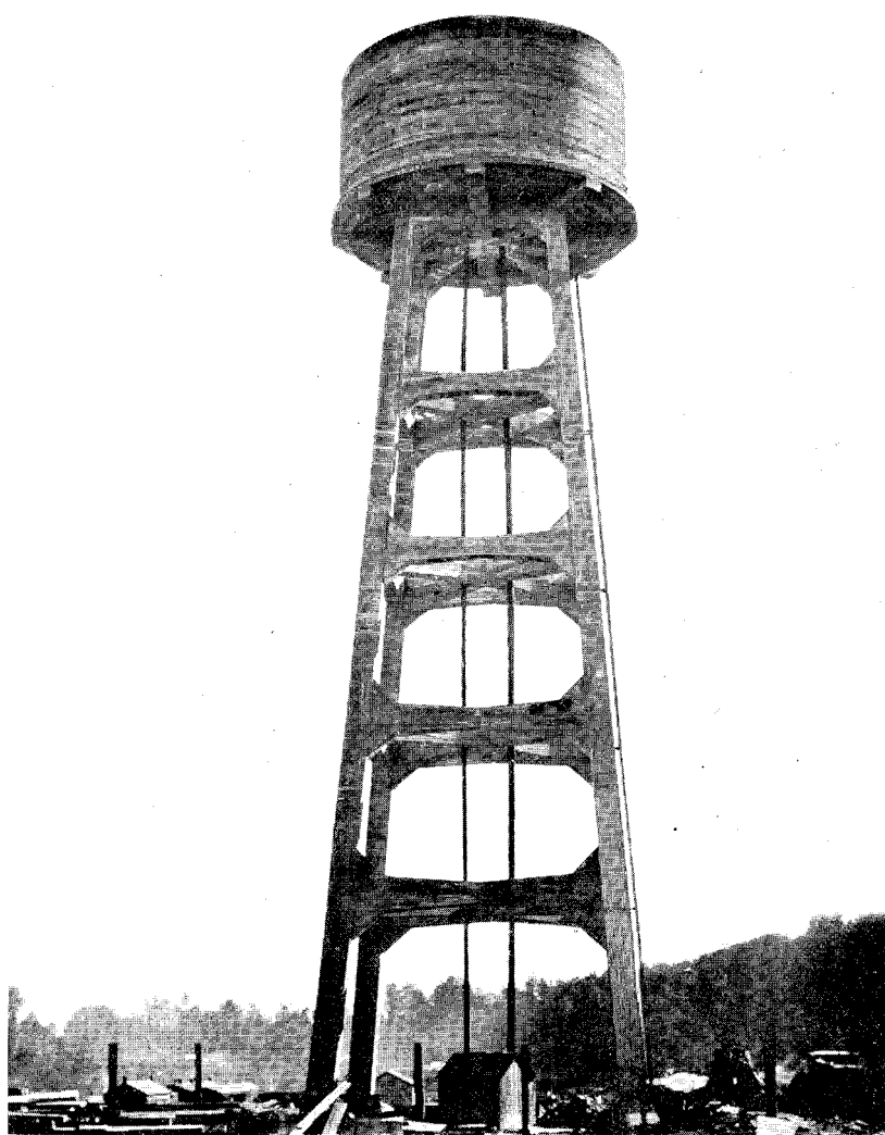
NORTH ISLAND MAIN TRUNK RAILWAY.— OHAKUNE STATION : FERRO-CONCRETE WATER-TANK AND TOWER.
