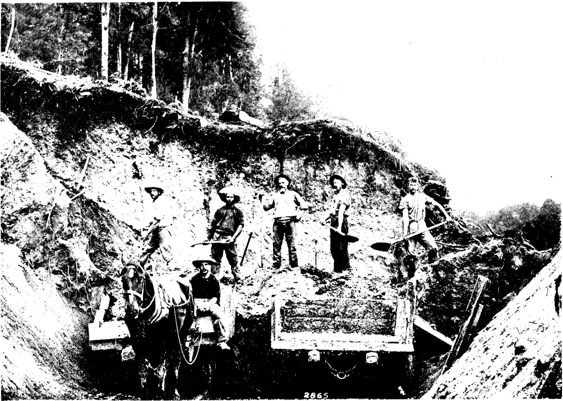
CO-OPERATIVE WORKMEN ON RAILWAY-CONSTRUCTION WORK.
