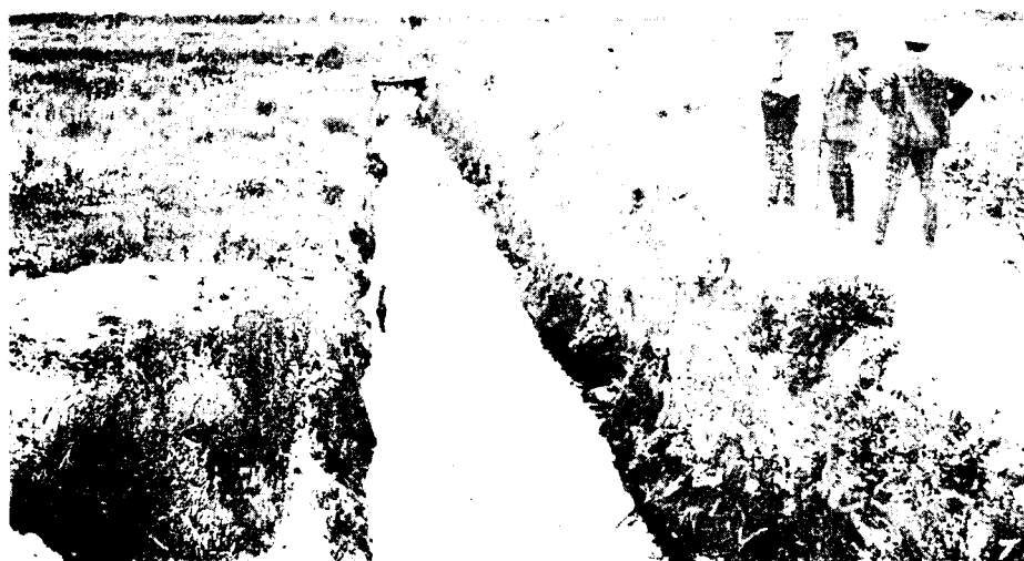
ONE OF THE DRAINS.
