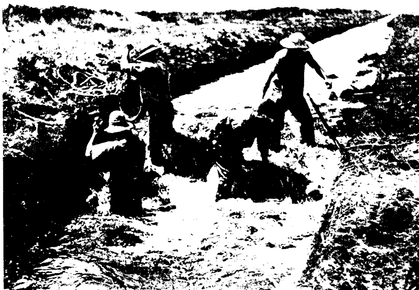
STRIPPING AND CLEARING DRAINS.
