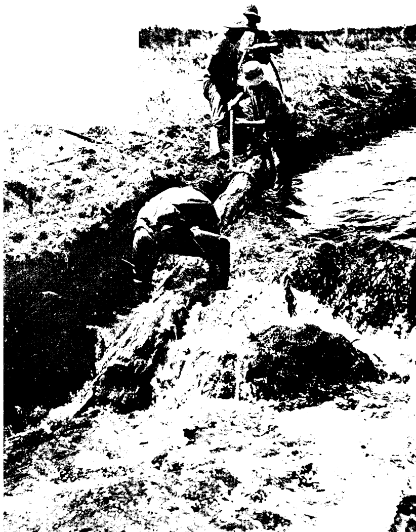
STRIPPING AND CLEARING DRAINS.
