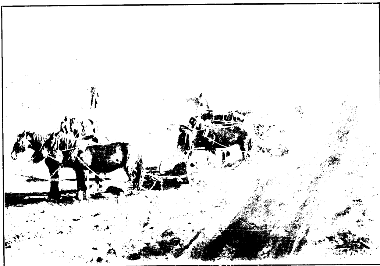
DRAYS AND SCOOPS ON ROAD FORMATION, WALLOA BLOCK.
