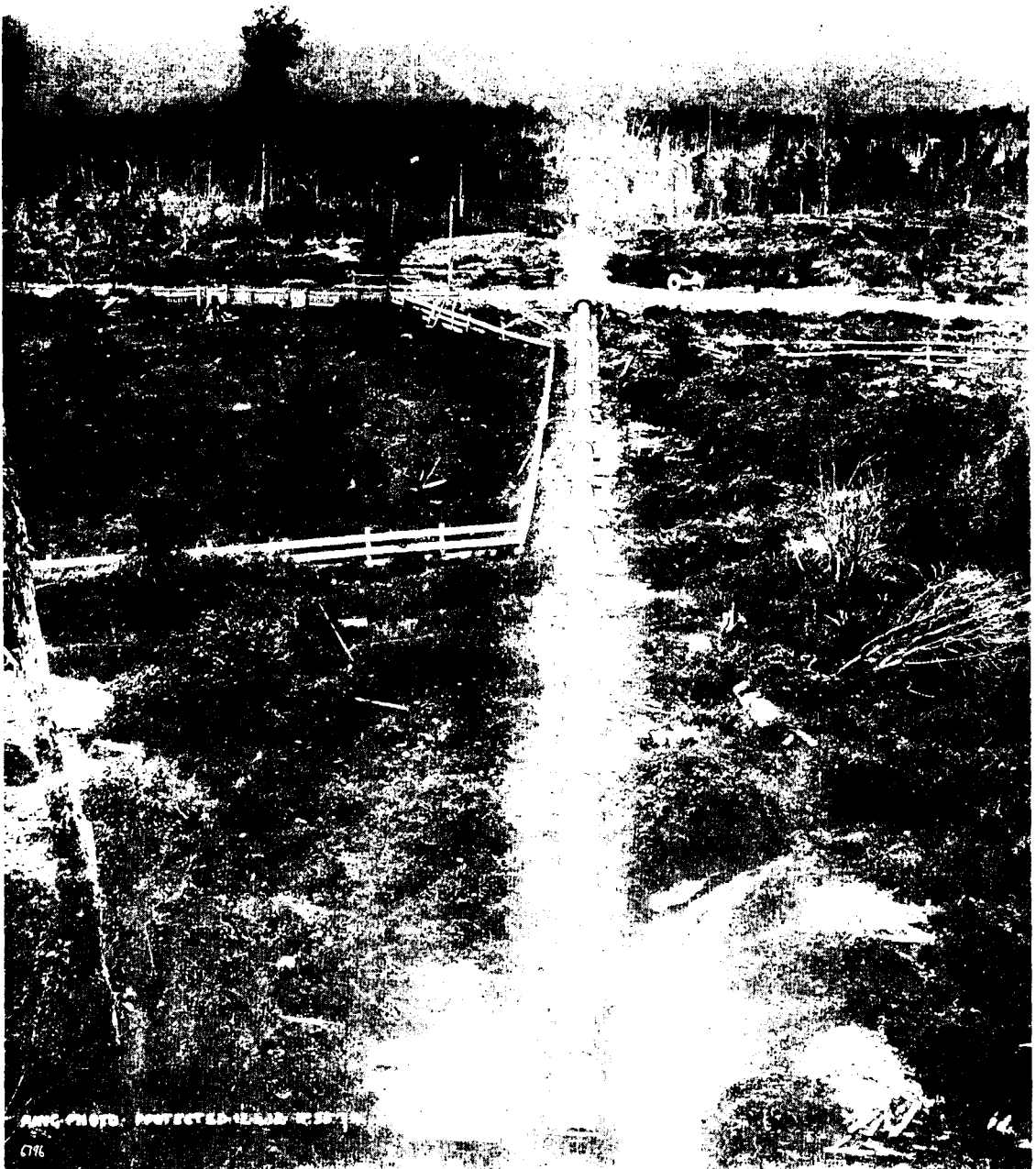
KUMAYA GOVERNMENT MINING WATER PACE EXTENSION. INVERTED SIPHON OF 30 INCH BORE, 2 MILES 1 CHAIN IN LENGTH, CROSSING THE VALLEY OF THE RIVER TARAMALAI, WESTLAND.
