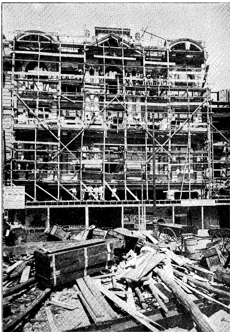
ILLUSTRATING SCAFFOLDING ERECTED UNDER THE SCAFFOLDING INSPECTION ACT, 1908.
