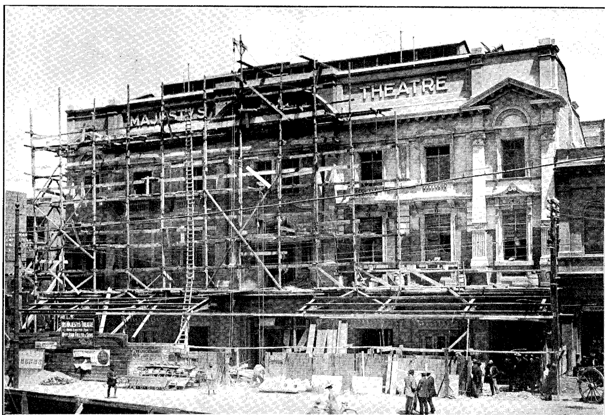
ILLUSTRATING SCAFFOLDING ERECTED UNDER THE SCAFFOLDING INSPECTION ACT, 1908.
