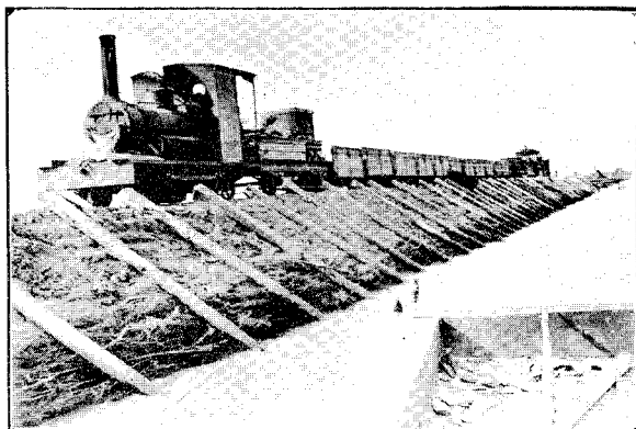
SECTION OF PRINCIPAL EMBANKMENT BEING CONSTRUCTED ON LINE OF OTATARA VIADUCT.
