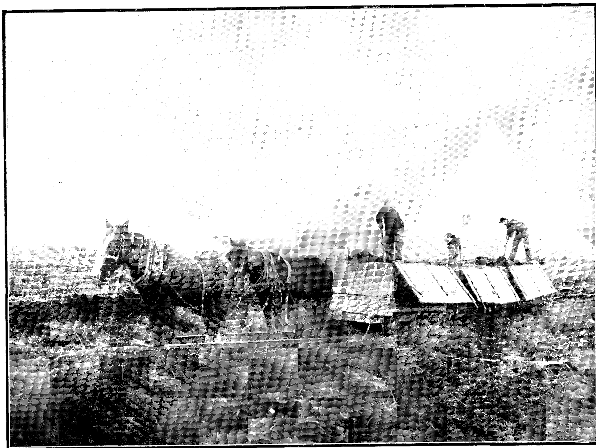
BALLASTING WAIKAKA TRAMWAY ROAD.
