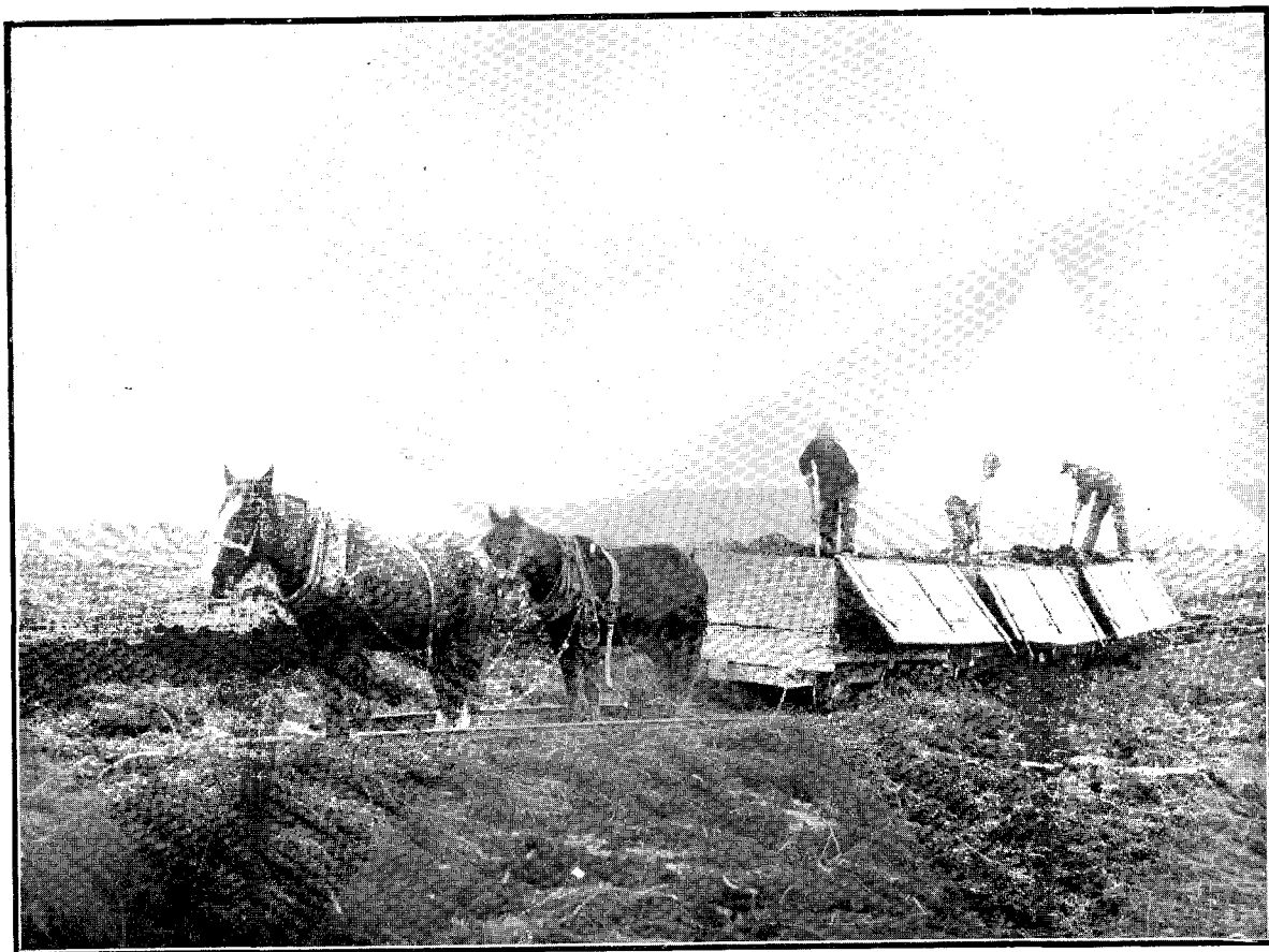
BALLASTING WAIKAKA TRAMWAY ROAD.
