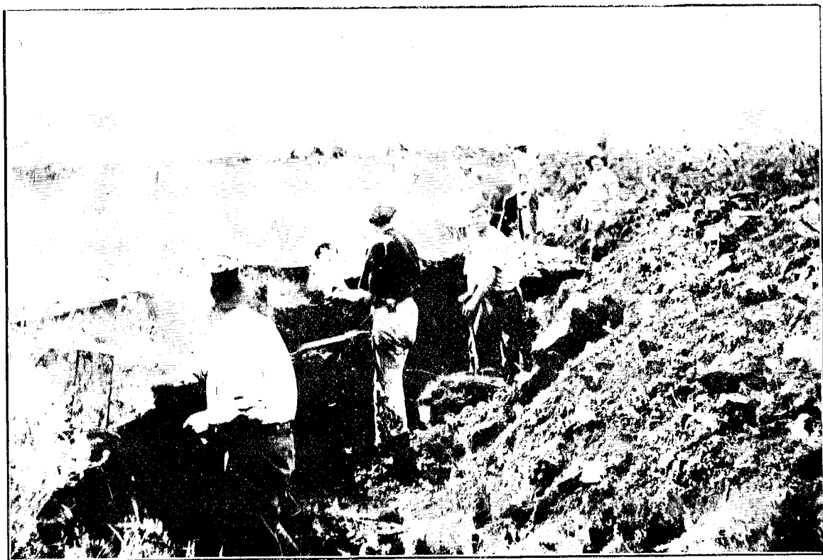
FACE DIGGING AT MANGAWAI.
