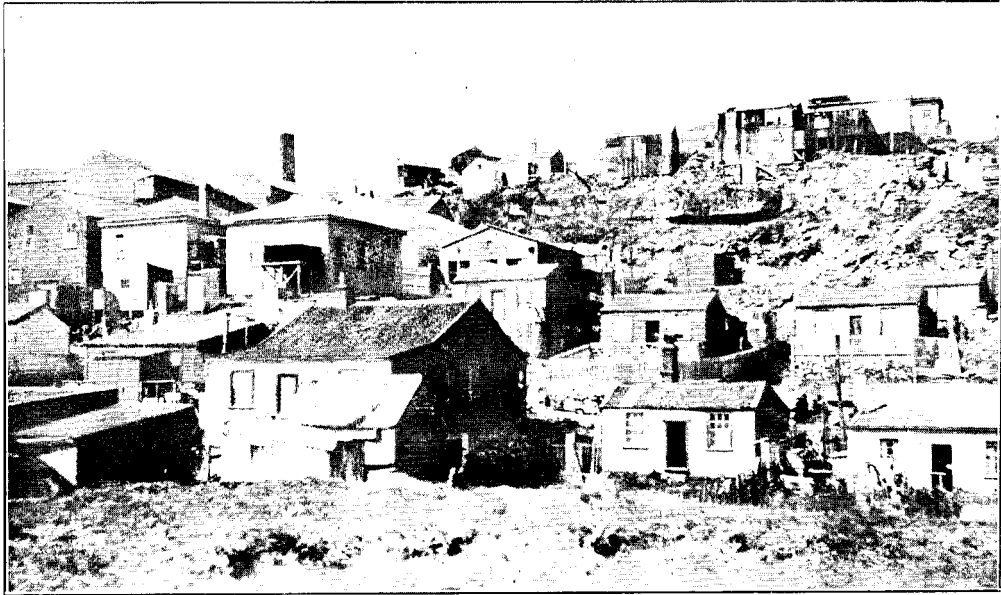
NO. 16. COLLECTION OF HUTS AND SHACKS ON WESTERN FACE OF DENNISTON HILL.
