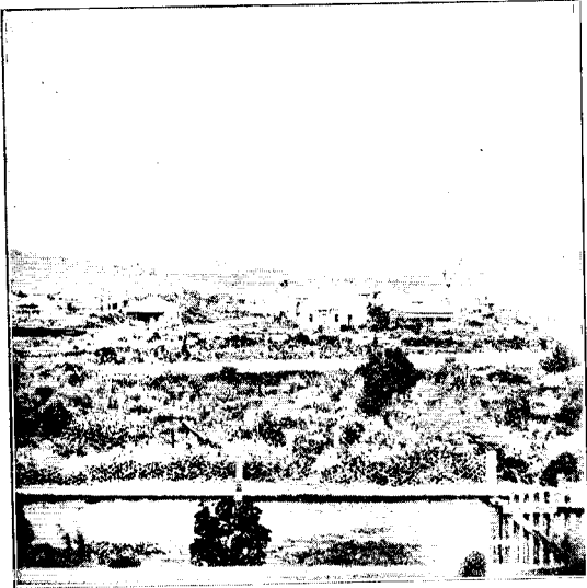
NO. 6. RUNANGA: GENERAL VIEW, SHOWING PRIVATELY OWNED HOMES AND THE MASONIC HALL.
