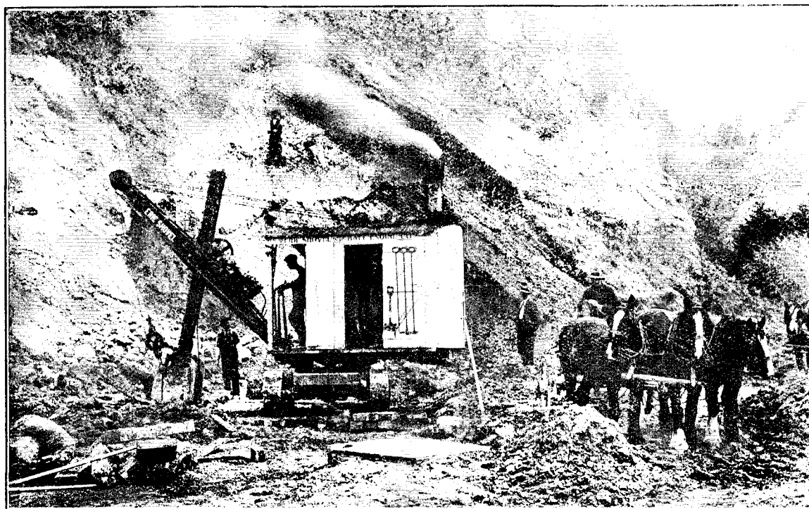
"ERIE" STEAM-SHOVEL AT WORK, HYDERABAD QUARRY, NAPIER.
