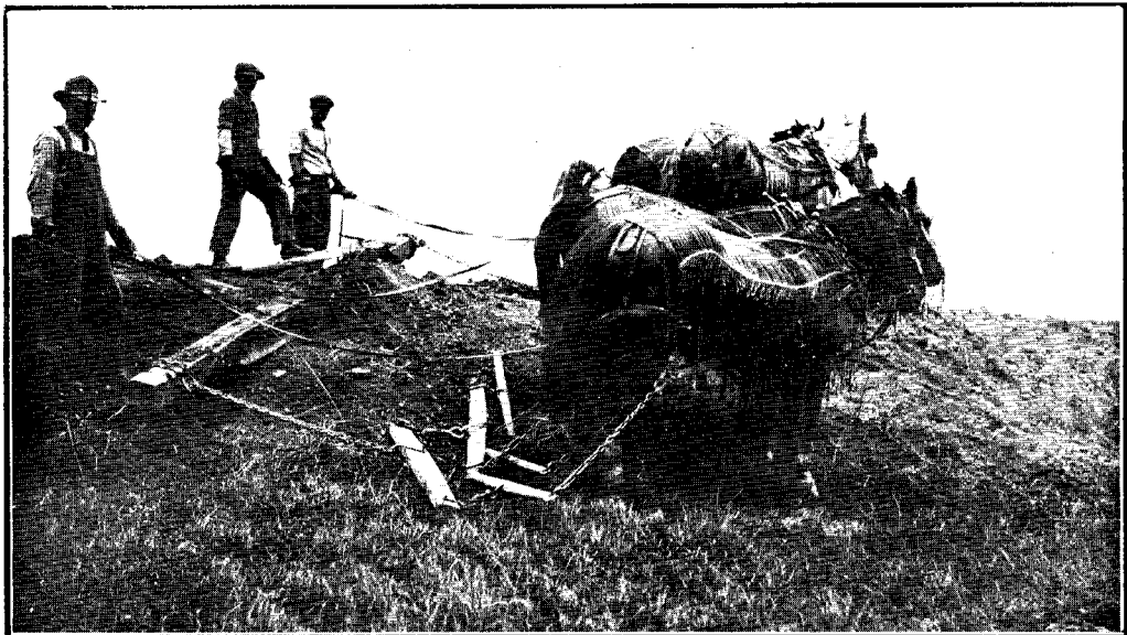
GRADING A SPOIL-BANK.
