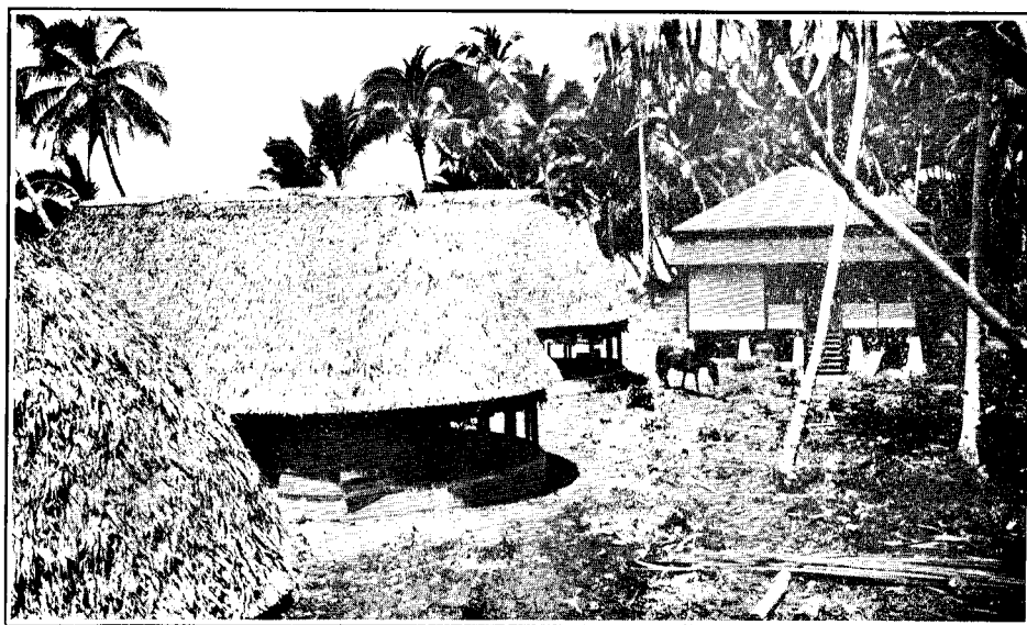
FIG. 11. District Hospital at Lalomann, in the Meipata district. This photograph was taken on completion of the buildings, before the grounds had been cleaned up.
