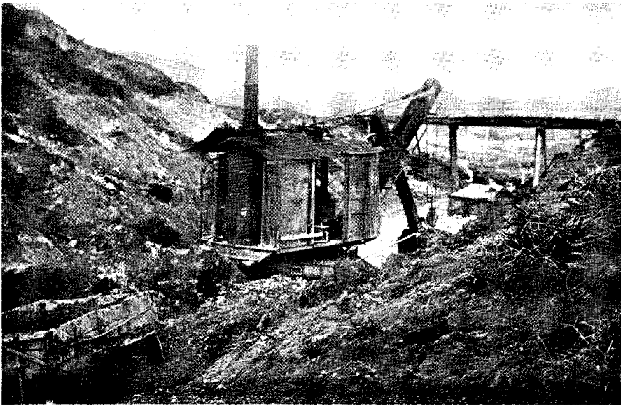
NORTH AUCKLAND MAIN TRUNK RAILWAY, KIRIKOPUNI SECTION. Steam-navvy at work.
