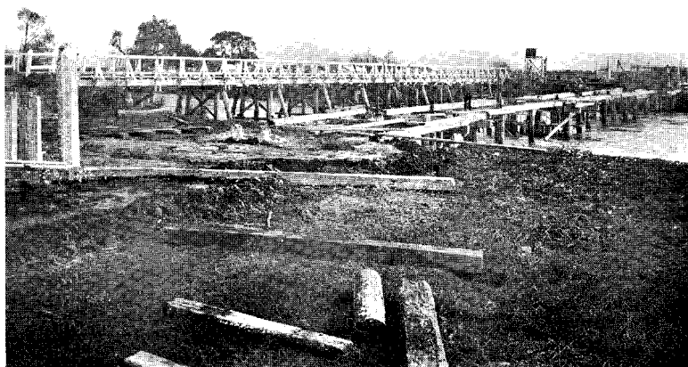
EAST COAST MAIN TRUNK RAILWAY, AWAKERI SECTION. Rangitaiki Bridge, at 87 m. 78 ch., under construction (temporary Road and Railway Bridge in background).
