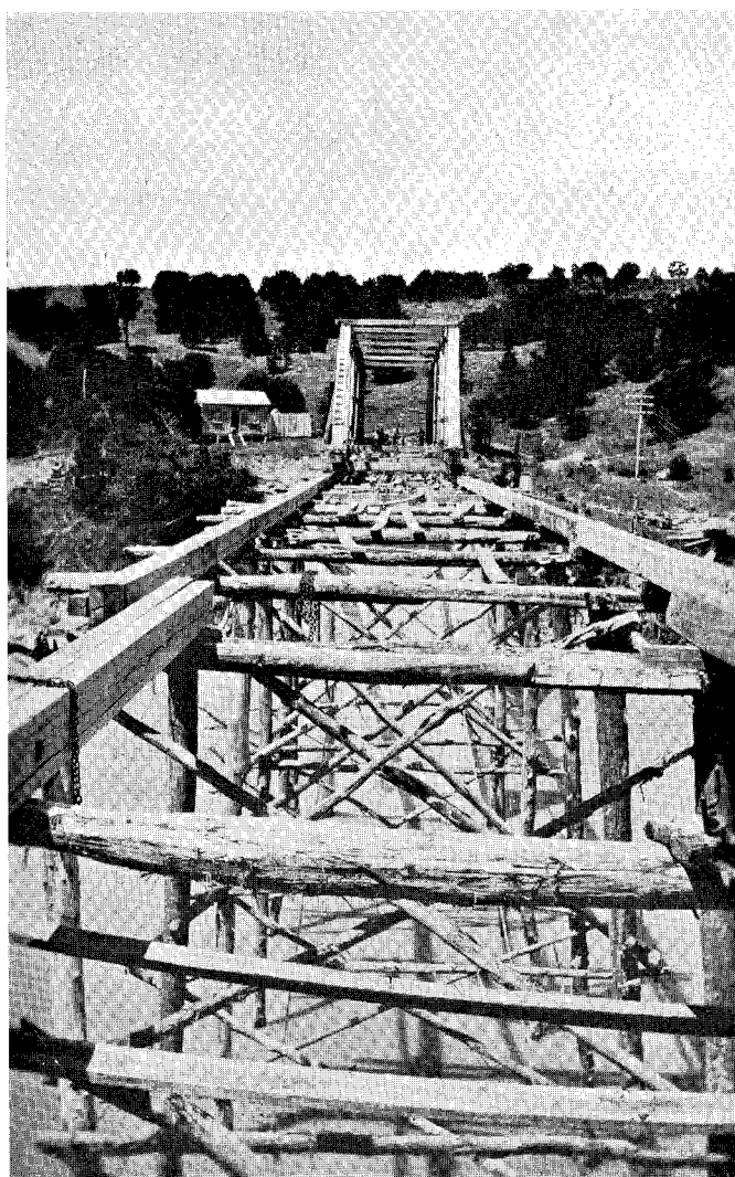
ROKOKAUTUKU BRIDGE UNDER CONSTRUCTION.
