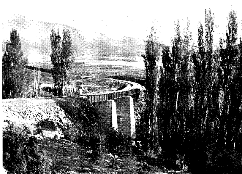
LAWRENCE-ROXBURGH RAILWAY. Minzion Burn Bridge.
