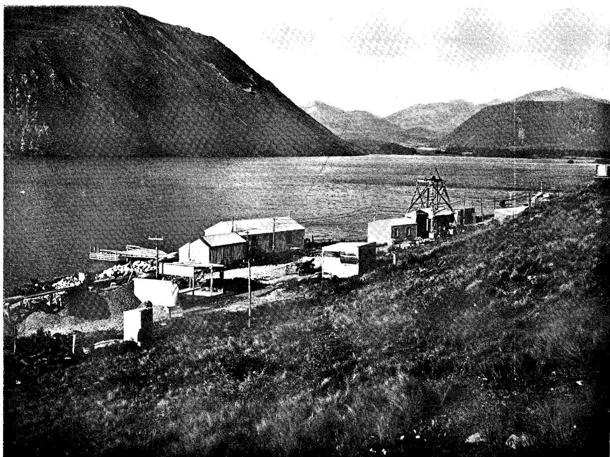
LAKE COLERIDGE HYDRO-ELECTRIC POWER PLANT. General view at Intake end of No. 2 Tunnel.
