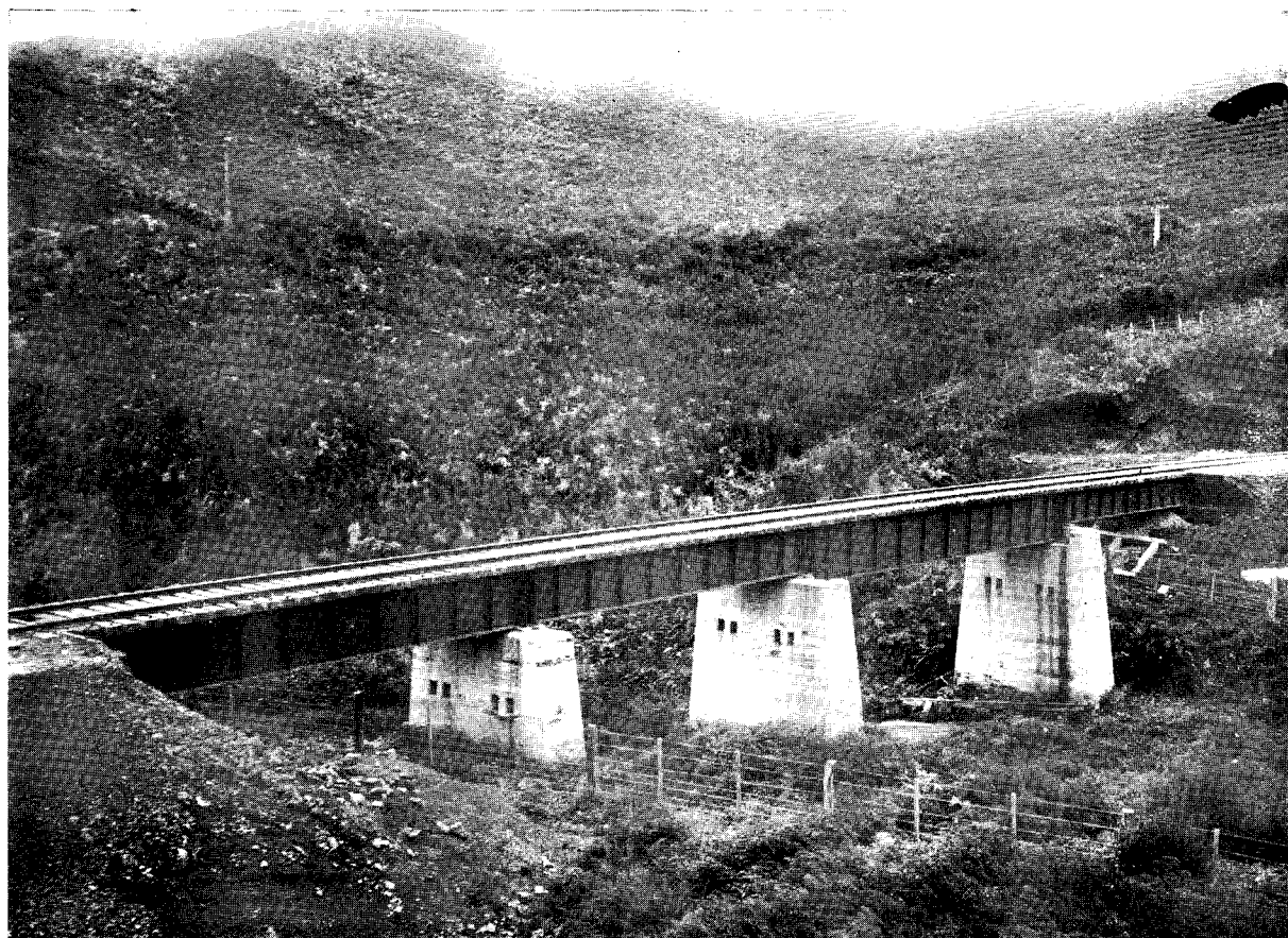
EAST COAST MAIN TRUNK RAILWAY, ATHENREE SECTION. Bridge at 7 m. 69 ch.
