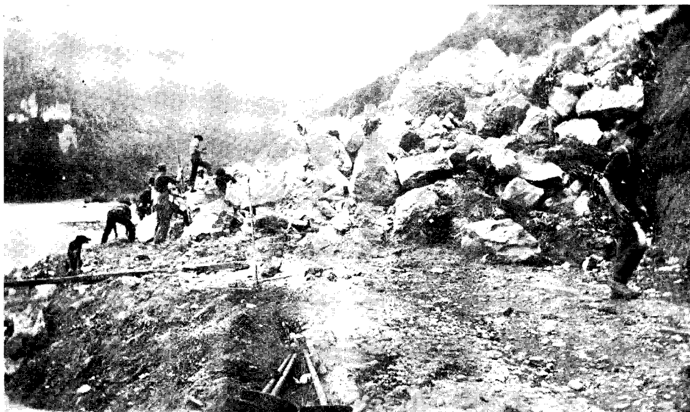
SLIP ON NELSON-WESTPORT HIGHWAY.
