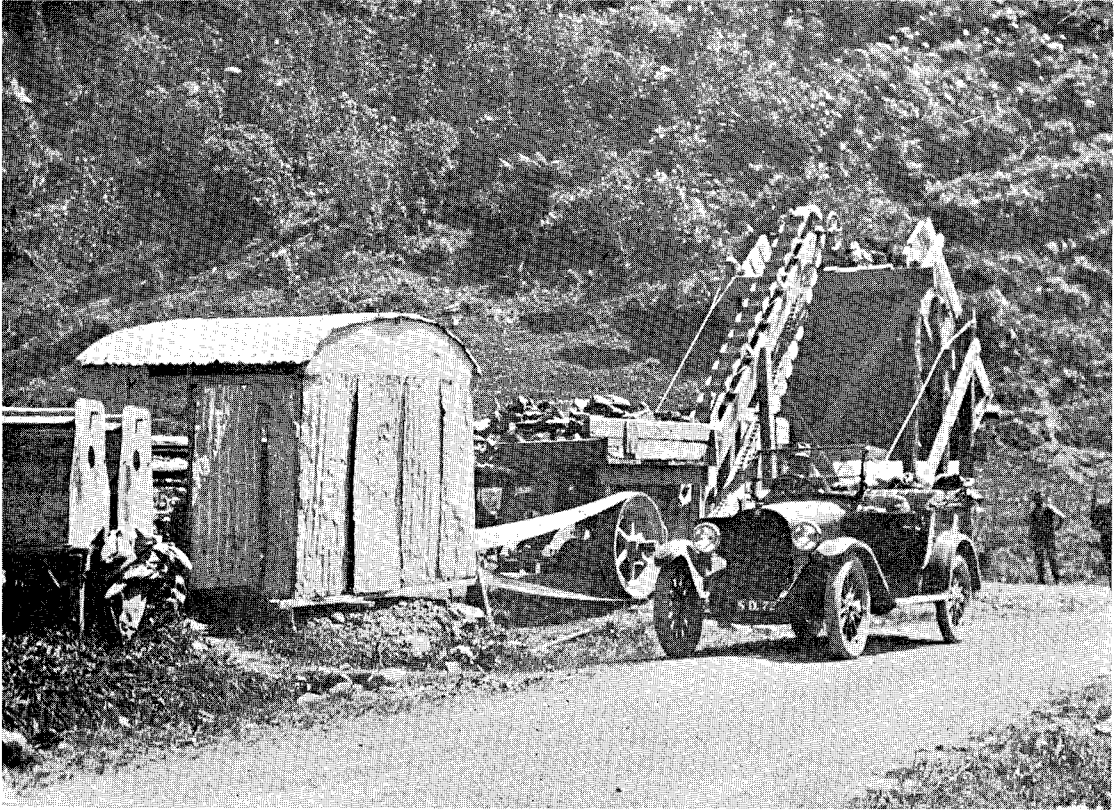
AUCKLAND—WELLINGTON (VIA TARANAKI) MAIN HIGHWAY. Lower Awakino Valley Road : Crushing Plant.
