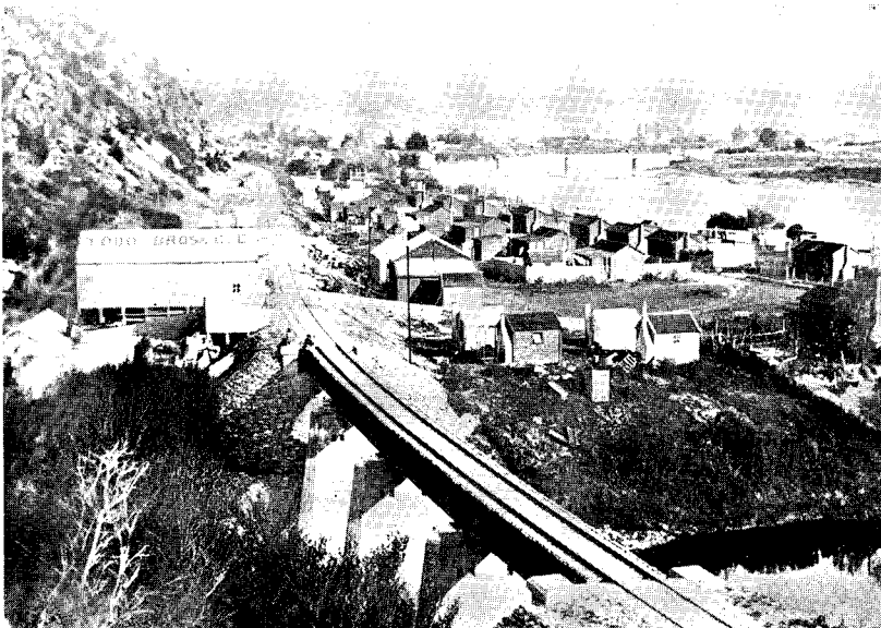
LAWRENCE-ROXBURGH RAILWAY. Beaumont River Bridge and Workmen's Camp.
