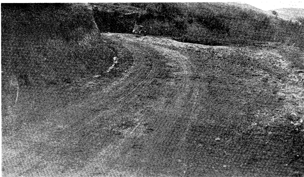
OTOKO HILL ROAD AFTER METALLING.
