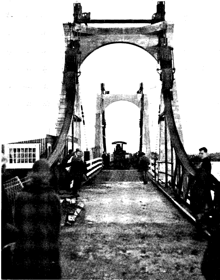
WAIROA RIVER ROAD-BRIDGE AT DARGAVILLE. Lift Span.
