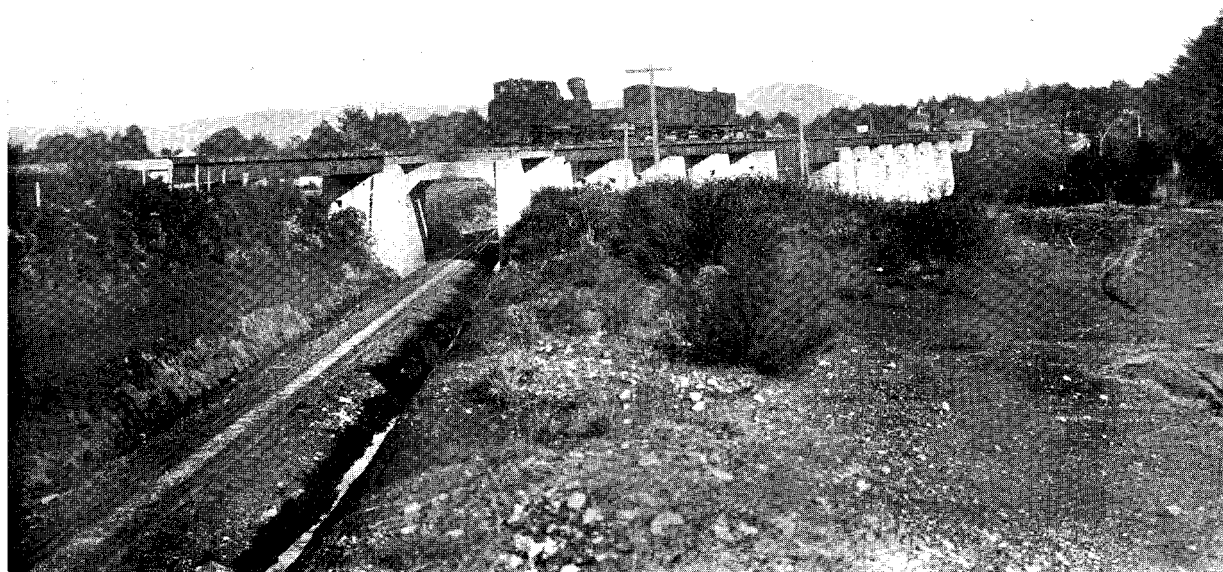
EAST COAST MAIN TRUNK RAILWAY, ATHENREE SECTION.
