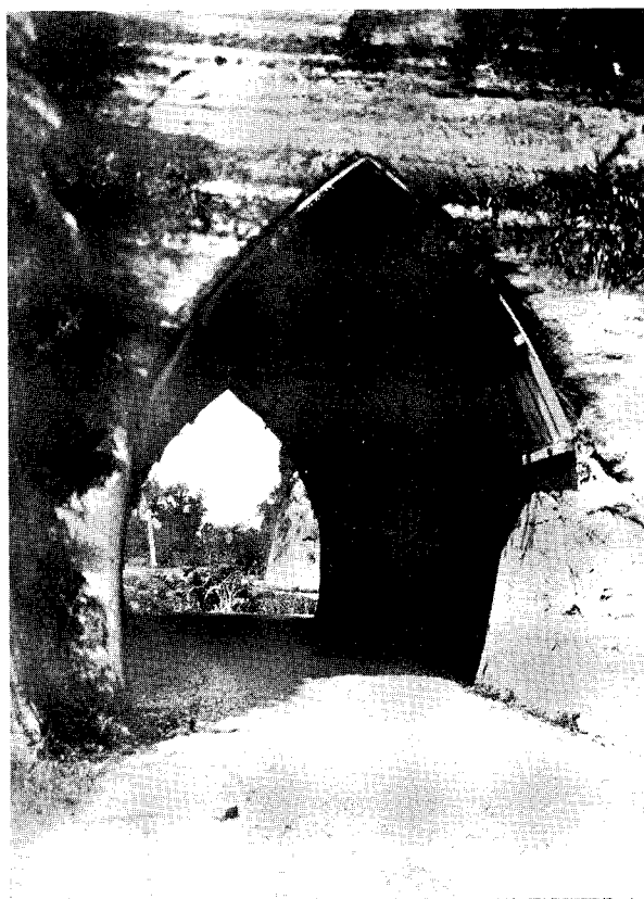
Road-tunnel, Mount Messenger.
