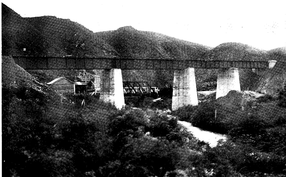
EAST COAST MAIN TRUNK RAILWAY, ATHENREE SECTION. Bridge at 70 m. 23 ch. (Quarry in background.)
