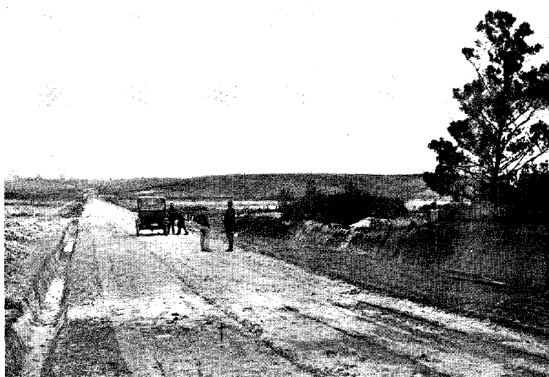
AUCKLAND-WELLINGTON (VIA TARANAKI) MAIN HIGHWAY. Rangiriri Deviation : Filling over Swamp at 3 m. 3 ch.
