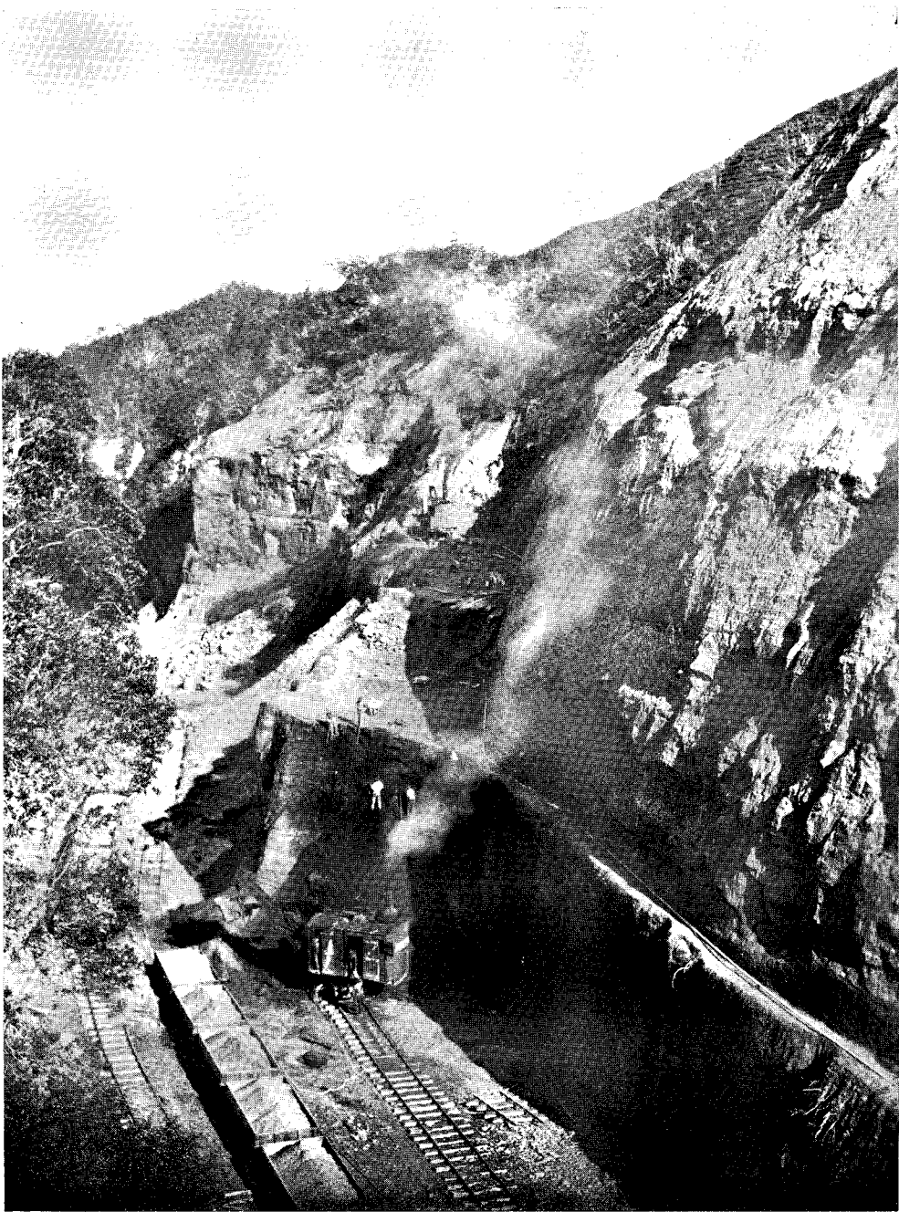
EAST COAST MAIN TRUNK RAILWAY, AWAKERI SECTION. Matata Quarry, at 79 m. 30 ch.: Steam-navvies at work stripping and loading.
