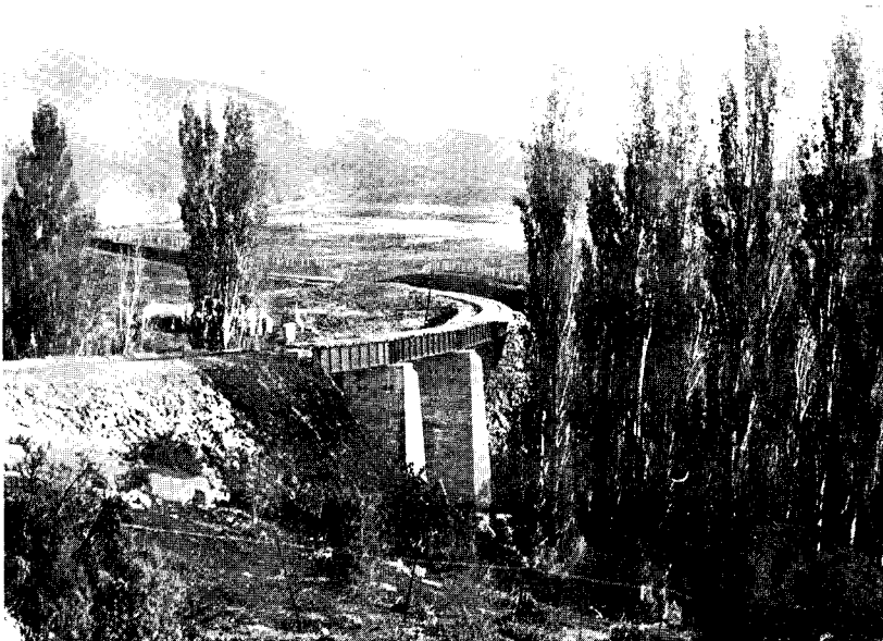
LAWRENCE-ROXBURGH RAILWAY. Minzion Burn Bridge.
