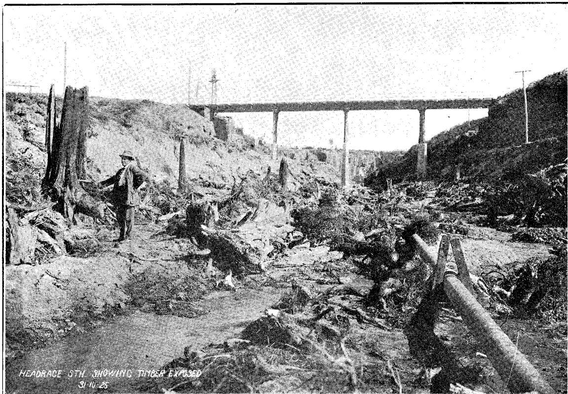
ARAPUNI HYDRO-ELECTRIC-POWER DEVELOPMENT: HEAD-RACE, SHOWING BURIED TIMBER.
