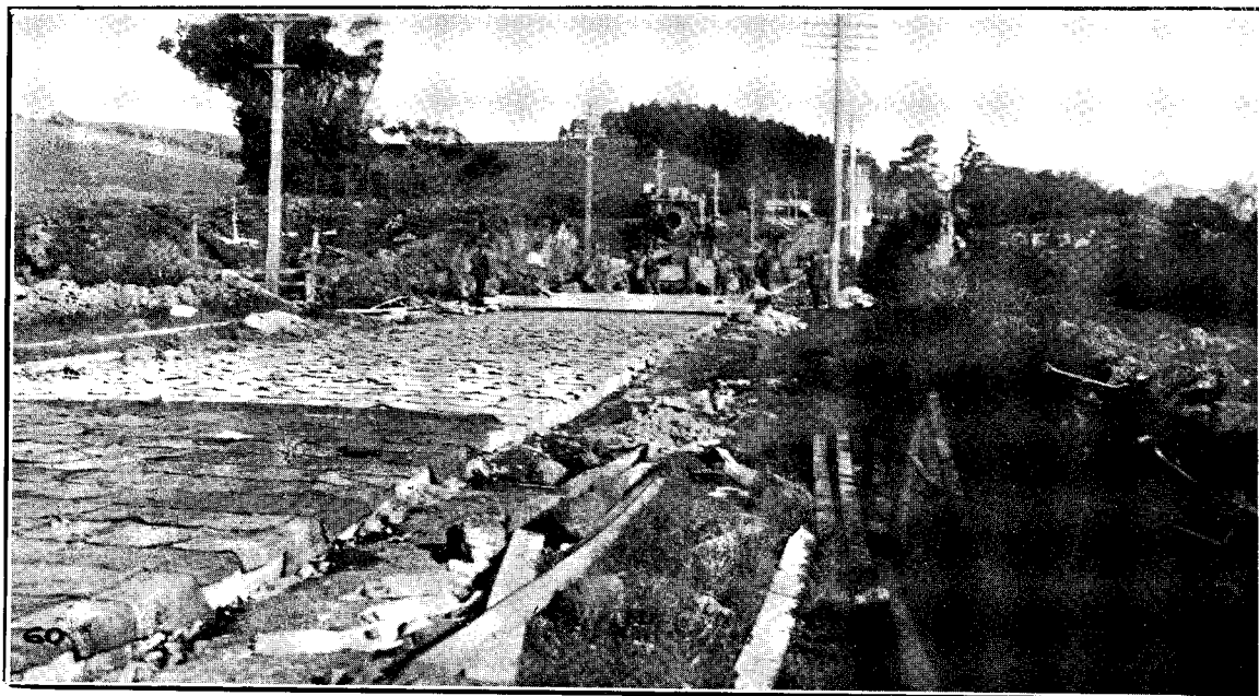
AUCKLAND-WELLINGTON (VIA TARANAKI) MAIN HIGHWAY, MOUNT WELLINGTON SECTION: CONCRETE PAVING IN PROGRESS.
