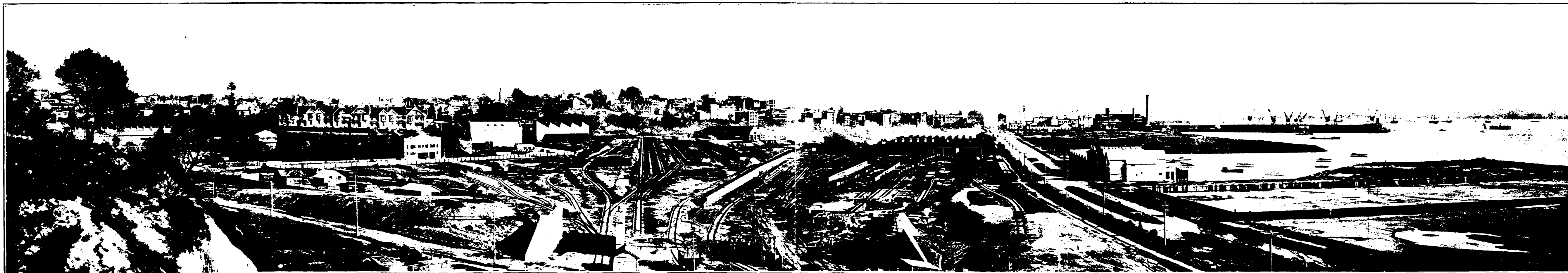
1926, SHOWING NEW STATION-YARD IN COURSE OF CONSTRUCTION.
