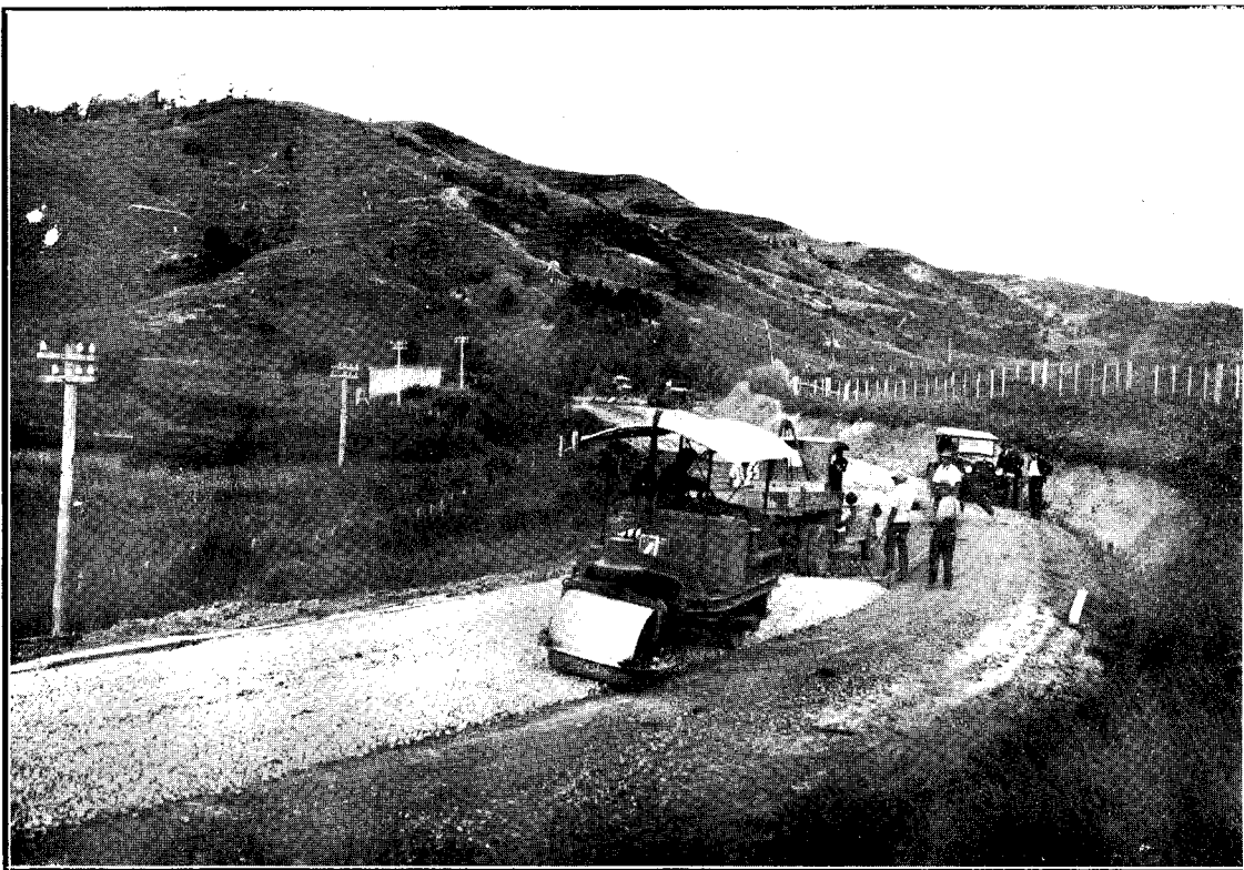
PLACING AND LOADING ROAD-METAL. KIRIKOPUNI-PARADISE ACCESS ROAD.
