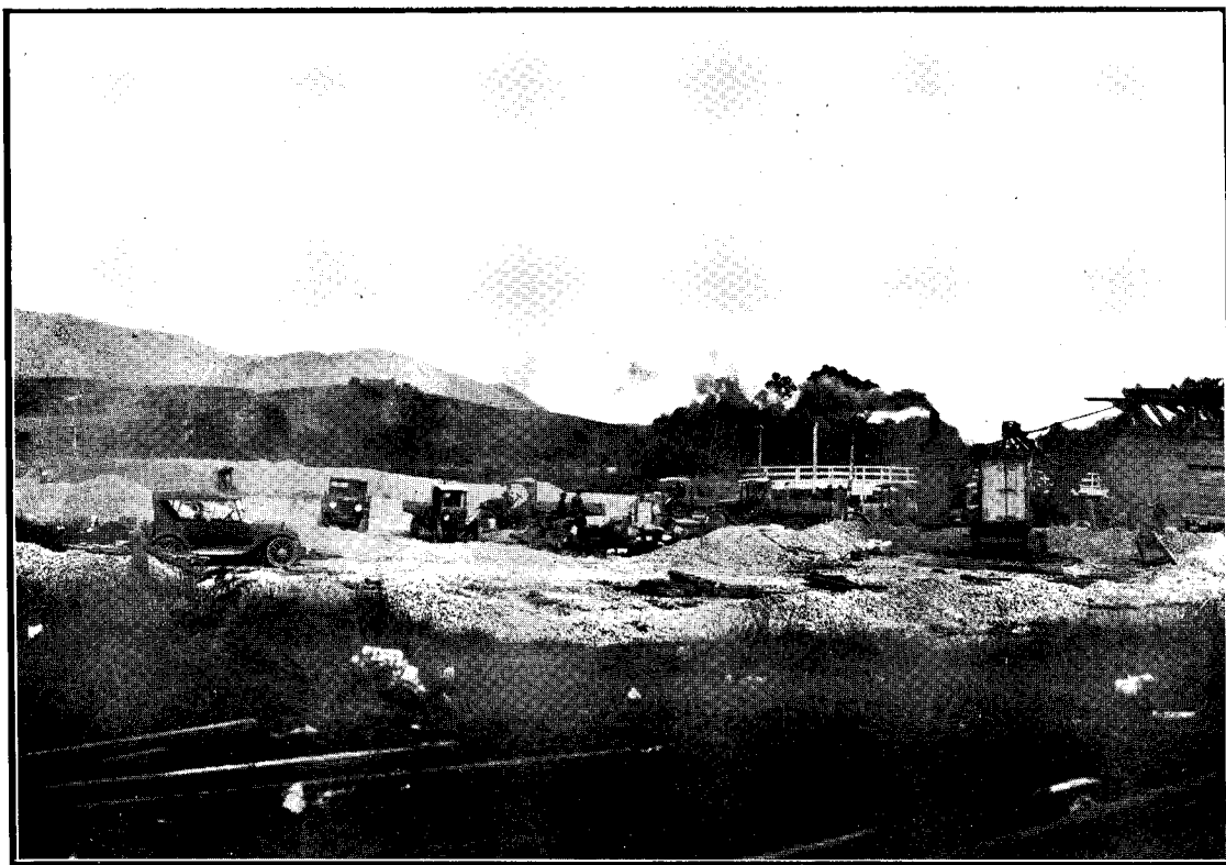
LOADING METAL AT KIRIKOPUNI. KIRIKOPUNI-PARAKAO ROAD.
