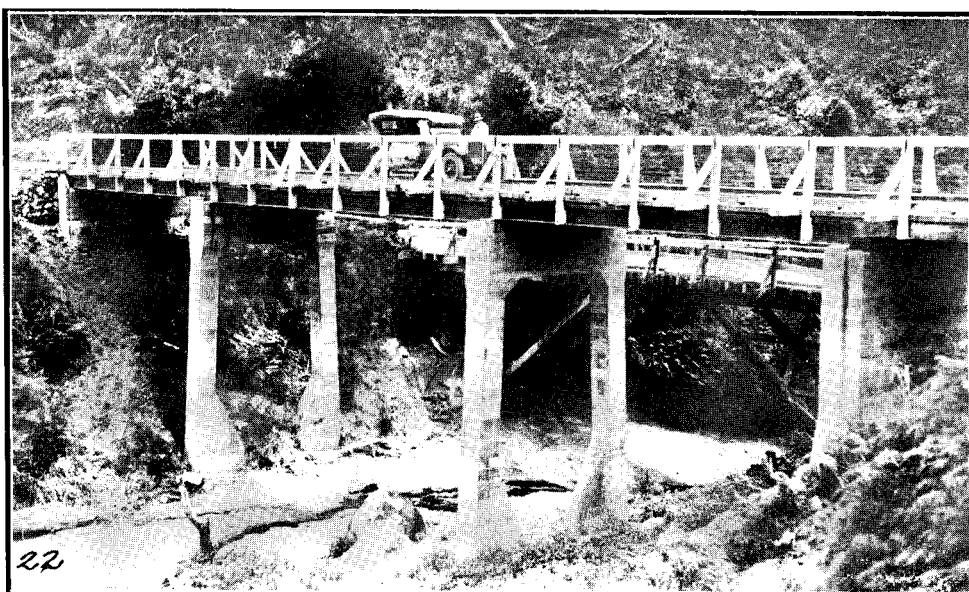
MANGAPOURI BRIDGE: ROLLED-STEEL JOISTS ON REINFORCED-CONCRETE PIERS. ROTORUA TAURANGA ROAD (DIRECT ROUTE).
