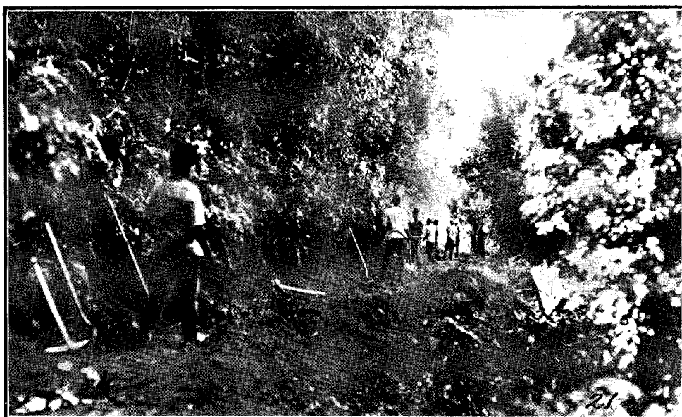
WIDENING ROAD TO DRAY-ROAD WIDTH. RUATAHUNA - WAIKAREMOANA ROAD.
