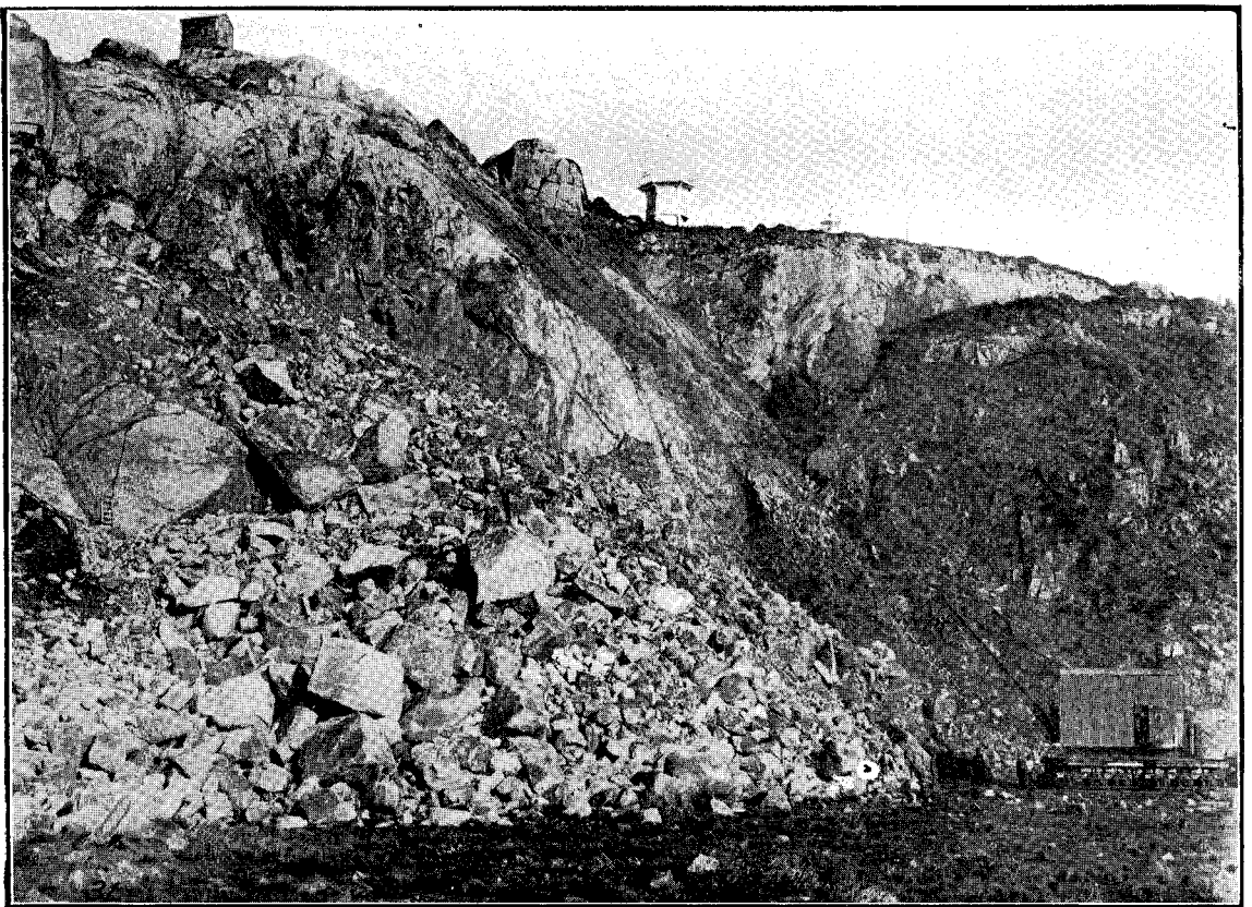
WESTPORT HARBOUR-WORKS: CAPE FOULWIND QUARRY.
