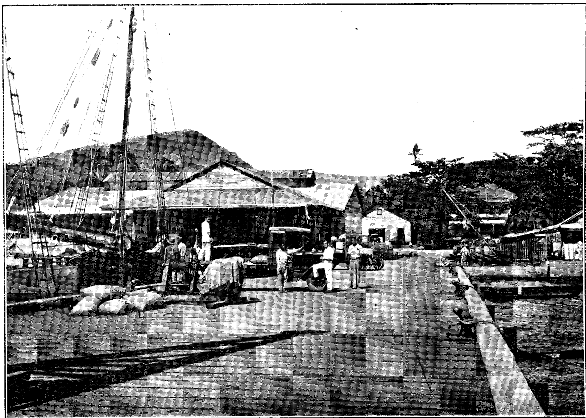
ANOTHER VIEW OF NEW CUSTOMS WHARF, APIA.
