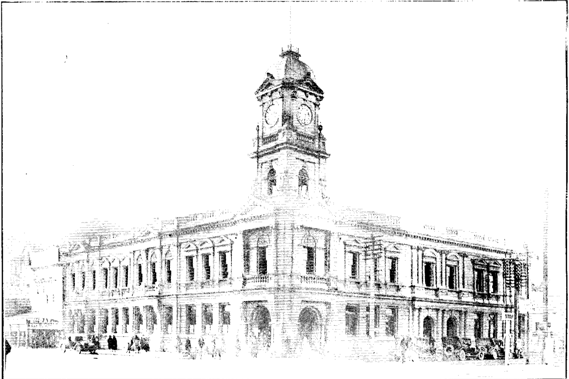
CHIEF POST-OFFICE BUILDING, PALMERSTON NORTH, TO WHICH AN EXTENSIVE ADDITION WAS MADE RECENTLY.
