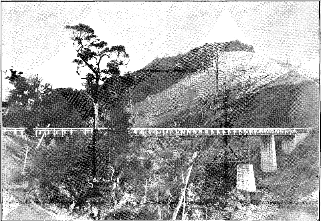
GENERAL ELEVATION OF BRIDGE. One 120 ft. steel truss and four 25 ft. timber spans.
