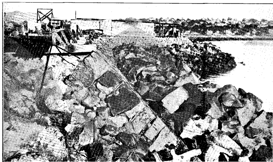
STONE PROTECTION WORK AT 2 M. 20 CH.
