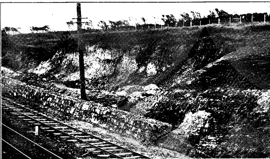
SLIP AT 5 M. 15 CH. AUCKLAND-WESTFIELD RAILWAY.
