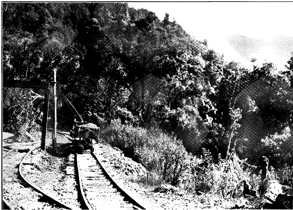
ELECTRIC LOCOMOTIVE MOVING SPOIL TO FILLING.
