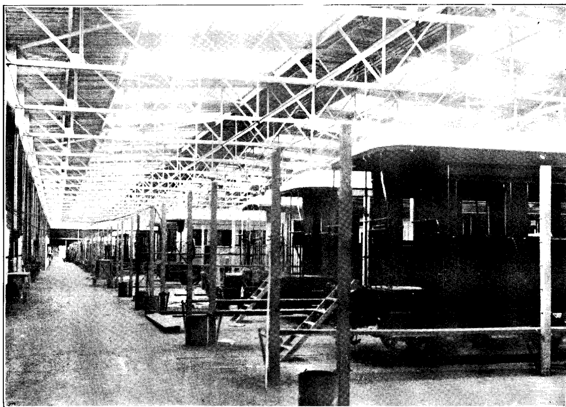
INTERIOR OF NO. 2 CAR SHOP, OTAHUHU.
