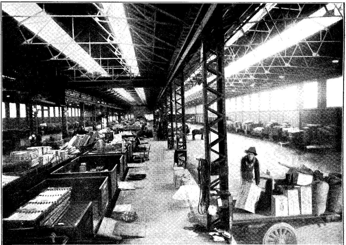
NEW OUTWARD-GOODS SHED, AUCKLAND.
