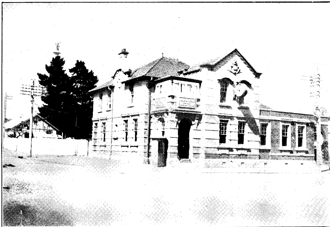
WAIPUKURAU POST-OFFICE BUILDING. (SHOWING RECENT ADDITION.)
