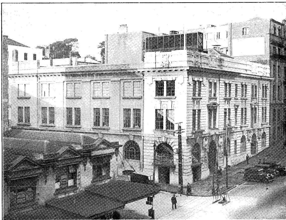
AUCKLAND: CENTRAL TELEPHONE EXCHANGE (INCLUDING RECENT ADDITION).
